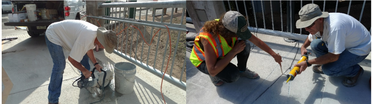
Figure 17. Example of Saw Cutting and Sealing Loops.
